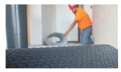
in multifamily construction where vinyl floor coverings allow applied loads to be passed directly through to the underlayment instead of being distributed over a larger area. Low deflection characteristics without sacrificing noise control, all in a low profile design.
